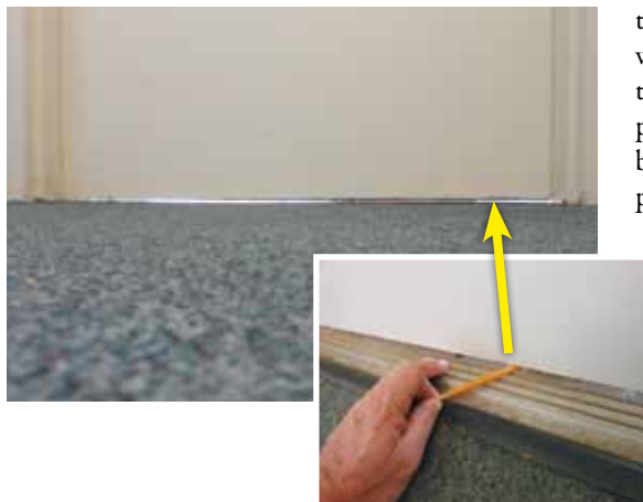
Figure 9. Crawling pests often enter structures by crawling under doors where gaps are present. The installation of a doorsweep can keep crawling invertebrates from inadvertently entering structures.
