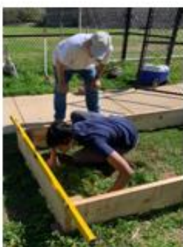
5. Leveling a raised bed.
