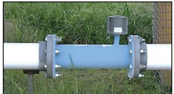
Figure 2. Position flow meter at the top of the line to ensure that water does not collect in the meter and is not susceptible to freezing.
